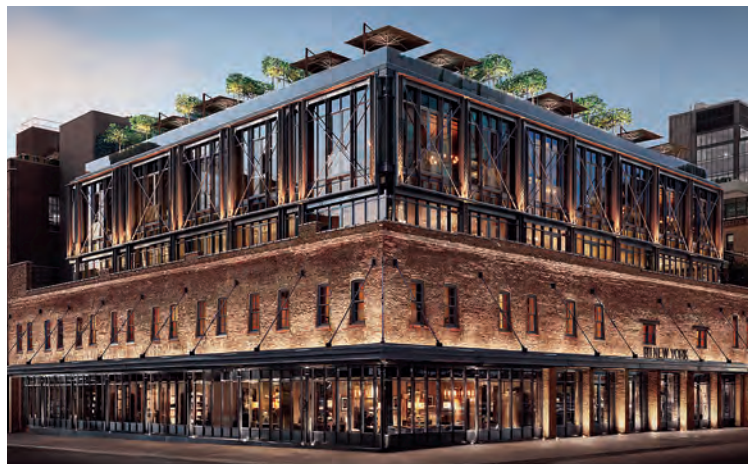
UP ON THE ROOF. The RH in New York's Meatpacking District has a rooftop restaurant, one of 16 restaurants the chain runs.
